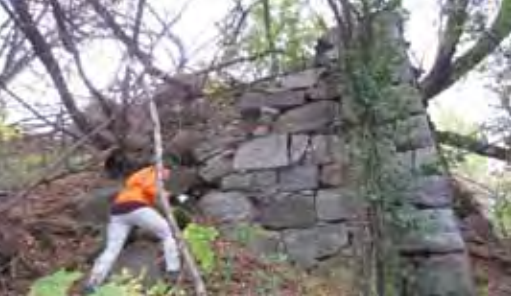
Elizabeth Lee leads tours around Westport. Here, she examines the Sisco Furnace ruin at Normandy Beach Club. Photograph by Virginia Westbrook.
