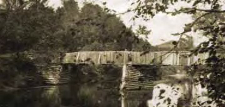
The dam broke in the spring of 1866, sending the contents of the mill pond over the falls and washing away the bridge at the foot of Church Street. At the time, a plank bridge connected the hamlet with the grist mill. Afterwards, that bridge was extended to the far shore, and this first crossing abandoned. Image courtesy of Evelyn Brant.
